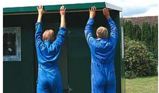
Fit the outer roof skin
