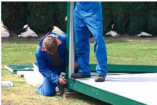
Fix the four corner posts
