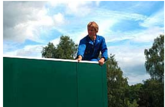
Fit the ceiling retention bars
