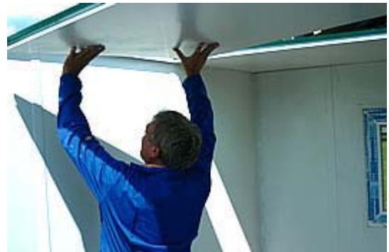
Slide in the ceiling panels
