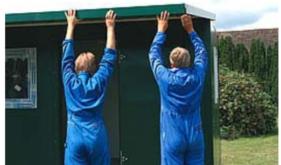
Fit the outer roof skin
