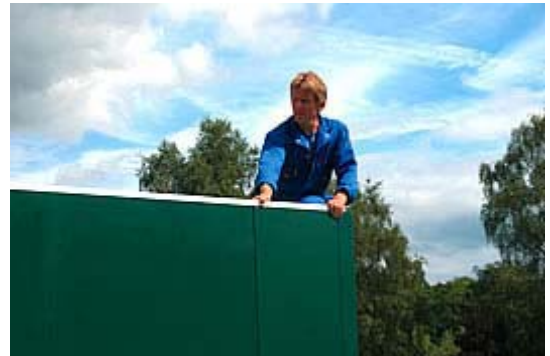
Fit the ceiling retention bars
