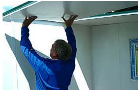
Slide in the ceiling panels
