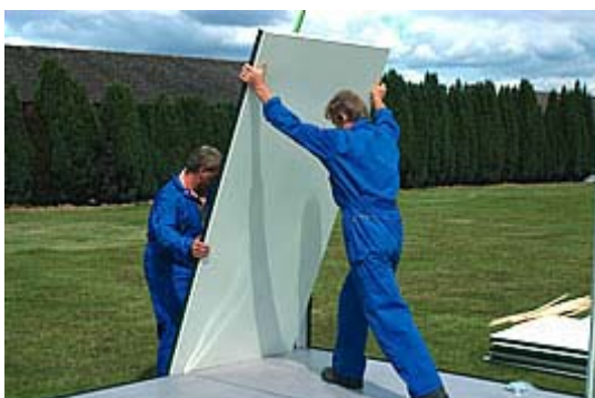
Slide in the wall, door & window panels
