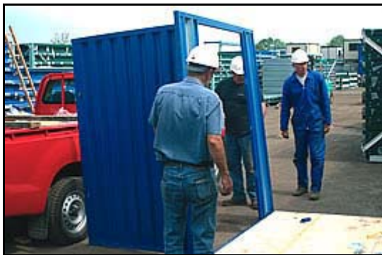
Attach the panels to the base of the unit
