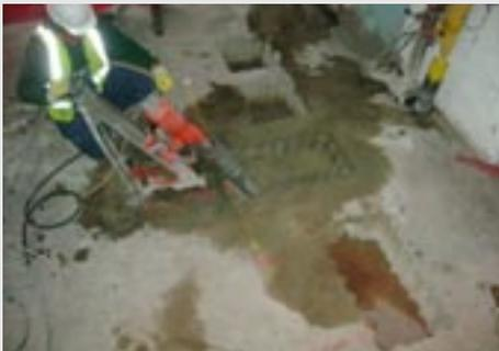
*Diamond Drill rig drills angled hole to form opening*
