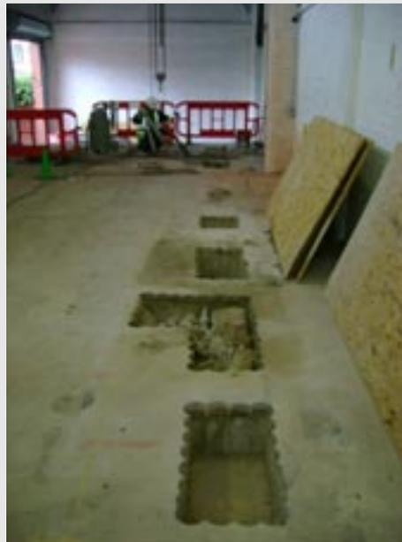
*Openings Stitch Diamond drilled in substation floorslab*
