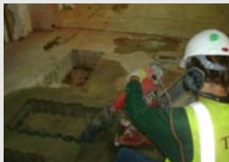
*Vibration and dust free drilling of opening for cable entry to electric substation*
