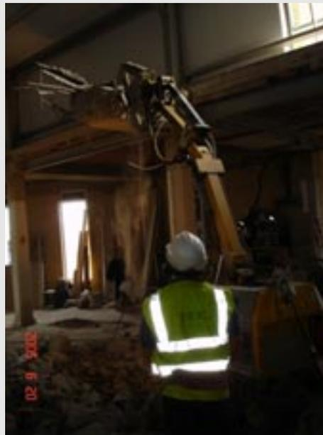
Robotic crusher breaks concrete structure to form opening without vibration and disruption to building occupiers
