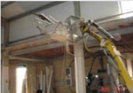
Demolition robot crushes reinforced concrete beam into rubble to form opening in floor slab
