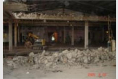
Brokk robot crushes large opening in roofslab to increase headroom of room
