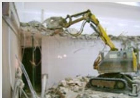
Brokk robot crushes out reinforced concrete floor in factory without disturbance to offices above
