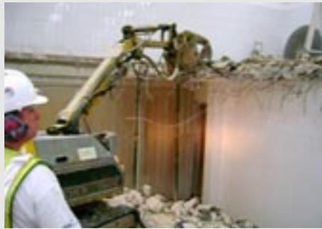
Hydraulic jaws on demolition robot crush out floor without noise or vibration.
