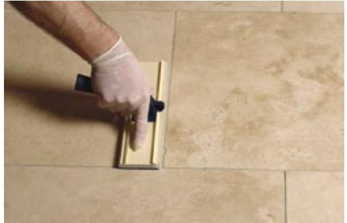
Apply a thin uniform coat of R R Stone Seal by sponge applicator, soft brush, cloth pad or spray until surface is wet ensuring that hollows and grout are covered. Rework over the areas that soak the sealant up quickly until the stone remains wet for at least 2-5 seconds.
