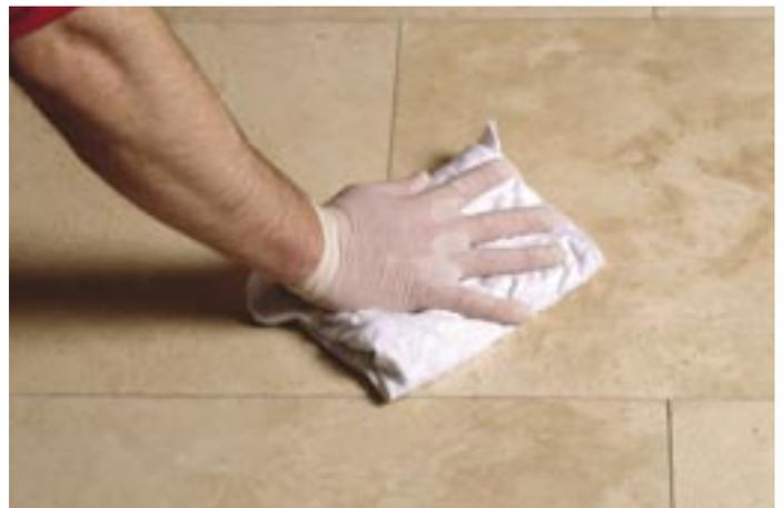
To remove the excess sealant and even the surface fold your cotton cloth into a pad and gently wipe the area so that any sealant lines disappear. Start at the edges and work inwards towards the middle.
