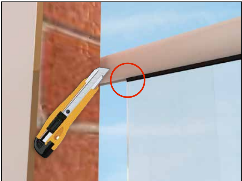
15. Trim off excess rubber.
