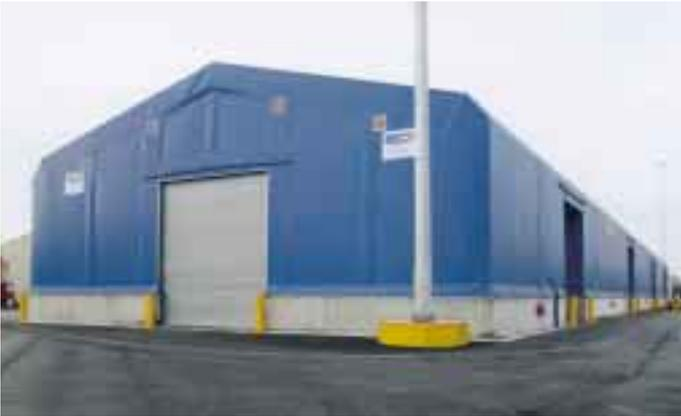
Dublin Port Company has become one of Rubb Buildings' latest export successes, with the purchase of a 32,390 sq.ft relocatable warehouse facility. Features include a 65.6x20' folding shutter door plus a further six 20x20' roller doors.
