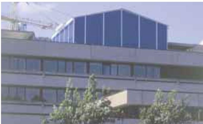
The Oasen Shopping Center in Bergen, needed to repair the roof of the main building. To be able to work under cover they erected a Rubb MCS retractable roof cover. The structure is fully crane liftable.
