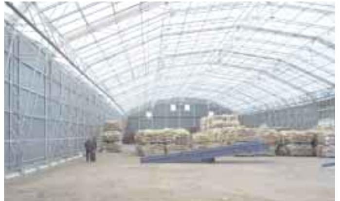
The Port required a facility that could be erected quickly in one location but relocated in the future to another site. Rubb provided an I-beam foundation that could be relocated along with the building.
