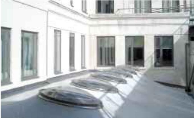
The challenge was to design and fabricate a roof for the school's unused courtyard to transform it into an atrium style cafe and meeting place. 23' x 100' and situated 4 stories up, the roof was fitted with polycarbonate domes which automatically open and close to suit environmental conditions.
