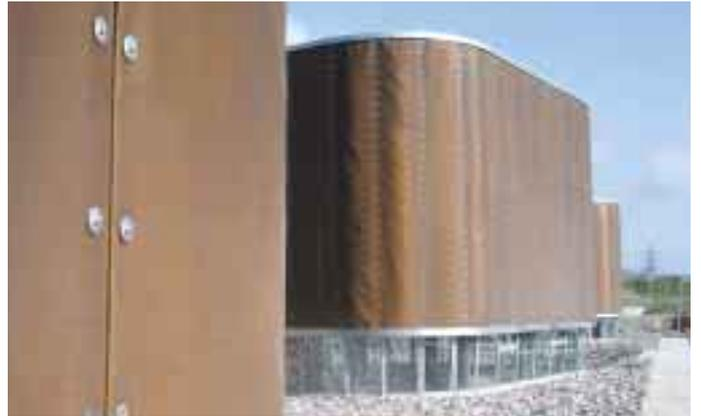
Bronze wire mesh rainscreen cladding was applied to exterior walls in the form of 26'x3' panels. High pressure water testing proved that the cladding exceeds British Standards for water tightness. It was recently one of the winners at the American Institute of Architects' London/UK Chapter 2003 design awards. Architect: Ian Ritchie Associates.
