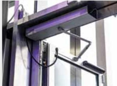
Two Slimdrive EMD-F electro-mechanical swing doors are fitted next to the revolving doors to provide easy access for those with mobility issues, they are opened using a press pad. The Slimdrive EMD-F operator is extremely discreet, at just 7cm high, and is exceptionally quiet in operation.
