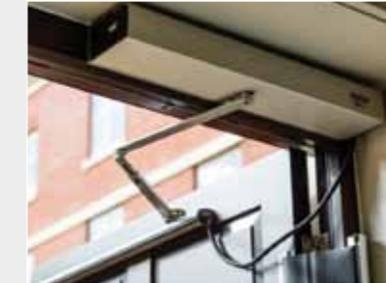
Inside over 2000 GEZE TS 2000 NV manual overhead door closers have been fitted to student rooms, corridors, and communal areas. Highly efficient with adjustable closing speed, hydraulic latching action and closing force, it features an over pressurisation valve which protects the internal workings of the units from damage.
