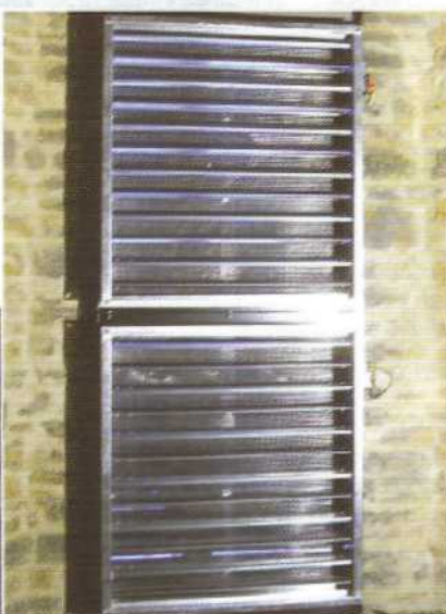
The finished louvres in the Minor's Tower
