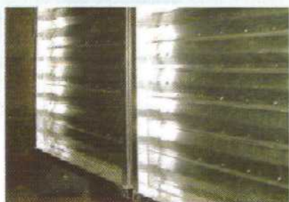
Dampers with fail-safe motors
