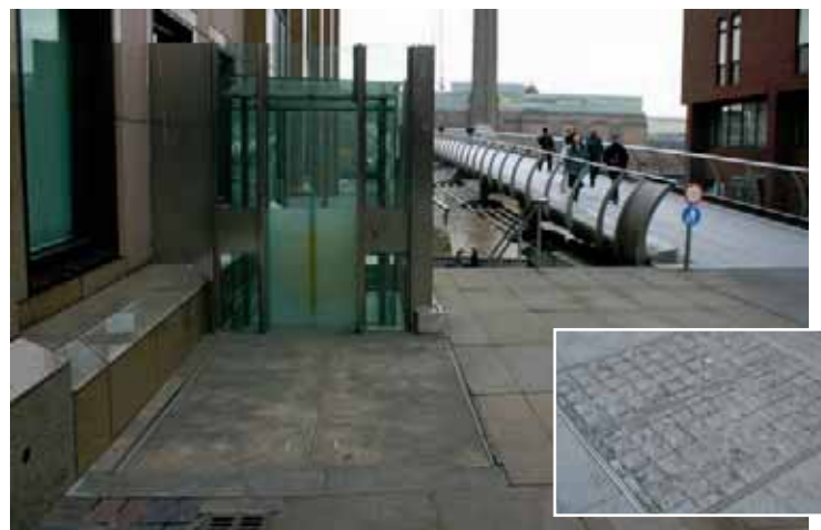
TER double leaf doors at Millennium Bridge London finished with a composite screed. Inset Bishops Square London TRD double leaf doors with brickwork infill
