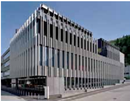
Corporate identity made visible. The vertical aluminium elements of the facade of the company's main office in Littau/Lucerne reflect Striebig's products and its relations with its market partners.
