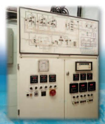
With the increasing levels of automation required by industry, AWE have continuously upgraded the type of control equipment which is used on automatic systems. Microprocessor controlled equipment is now available for the whole range of equipment, from the domestic softener to the large demineralisation plant. On the large custom designed plants, AWE work closely with the client, utilising the client's choice of microprocessor.
