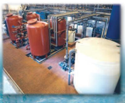
Dealkalisers use weak cation resin to convert the bicarbonates (alkalinity) in the water to carbonic acid. To remove the carbonic acid, the water is passed through a degasser tower. When exhausted, the resin is regenerated using acid.
