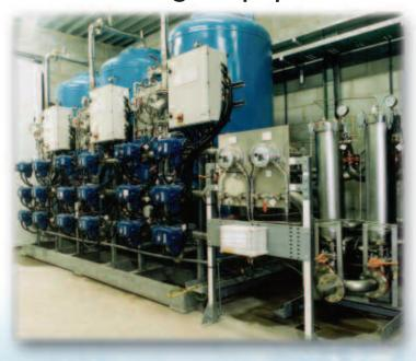
Ion Exchange forms the basis of several types of treatment which although utilising very similar equipment, by the use of different resins and chemicals, produces very different quality waters.
