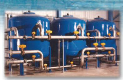
Backwashing is carried out by reversing the flow through the bed, thus lifting and expanding the filter bed. The grains of sand collide with each other and, in doing so, free the accumulated suspended solids which are swept away to drain with the backwash water. Sometimes air is injected prior to backwash water to break up the bed. This reduces the flow rate of backwash water required to effectively clean the filter bed.
