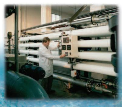
Reverse Osmosis is now an accepted and field tested process for the removal of both ionisable and non-ionisable impurities from water and other liquids, utilising hollow fibre or spiral wound modules. Units can be custom designed to suit all raw water conditions and capacities.
