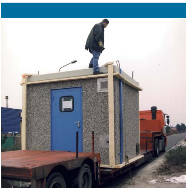
Pre-packaged water monitoring station
