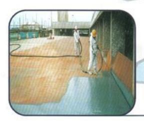
Euroshield cold applied liquid membrane, manufactured using synthetic resin solution is modified with polymeric fibres and bitumen. For waterproofing of surfaces with a minimum of preparation including metal, concrete, gutters, pipework is guaranteed for 10 and 15 years. 15 year guarantee system only if applied by an approved contractor.
