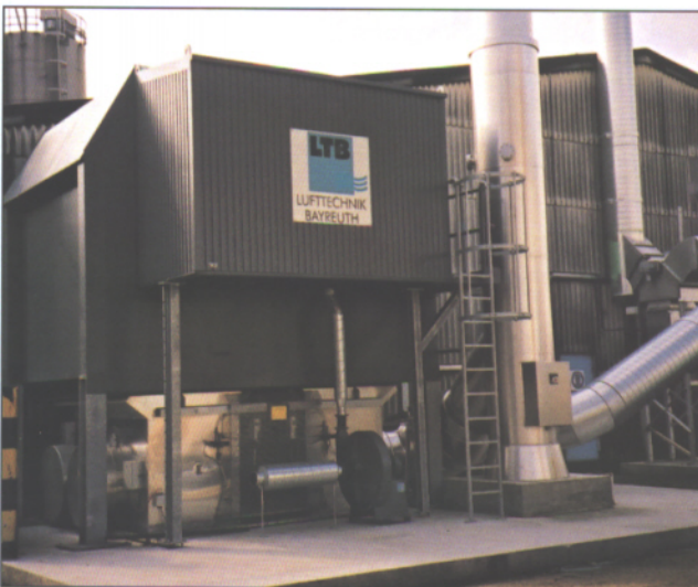
Roxitherm RTM 2-Chamber Oxidiser on Rotogravure Printing.
