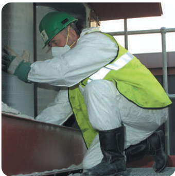
Filter Unit Servicing
