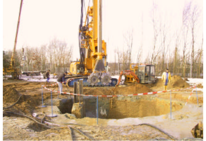
CSM rig on BG 22H, foreground: excavated test pit (dia. 8 m, wall depth 20 m)
