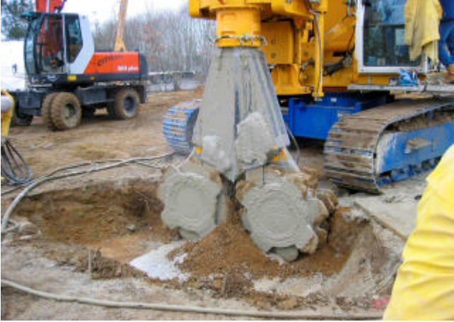
Setting-up of CSM tool at new location
