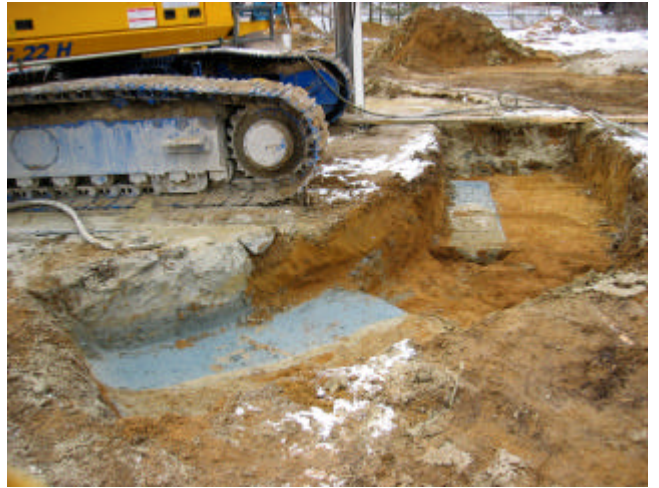
CSM rig on BG 22H, foreground: excavated test pit (dia. 8 m, wall depth 20 m)
