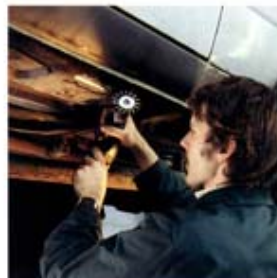
Removing under seal with a ultra shaft mounted circular brush.
