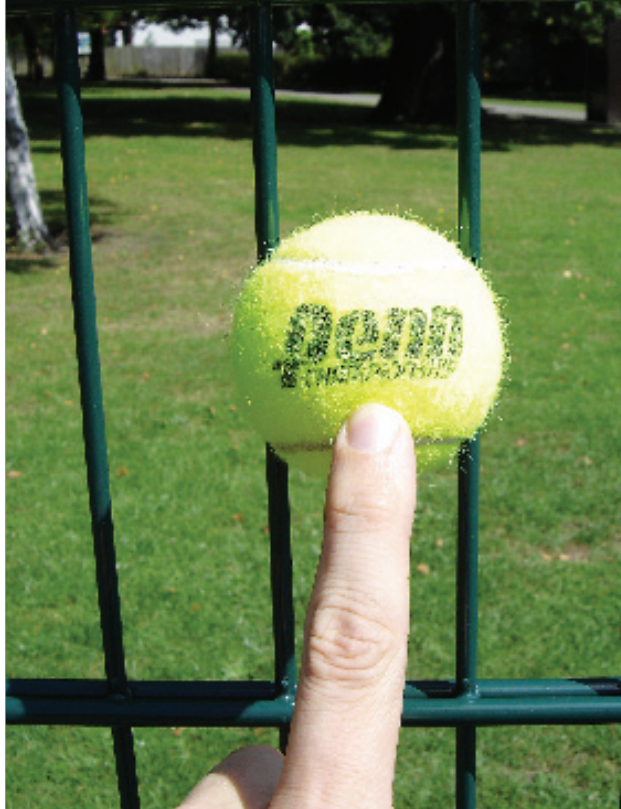
50mm Duo mesh Balls can deform and pass through the mesh
