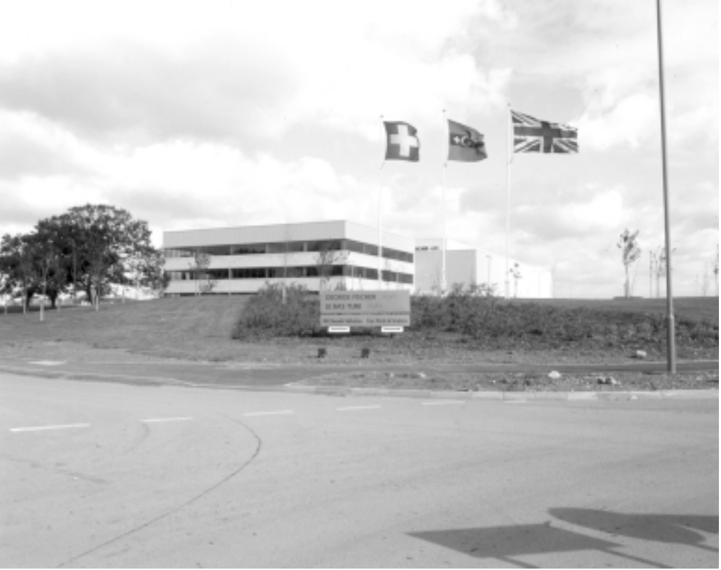
George Fischer Distribution Centre Coventry (DCC)
