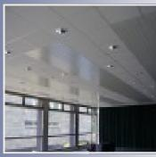
Wings Ecoline is Lightweight radiant heating panels consisting of an arrangement of 15 mm copper waterway tubes with 28mm headers. The tubes are pressed into aluminium profiles, streamline butt welded and soldered to ensure maximum contact between the aluminium profiles to create efficient heat transference to the faceplate.
