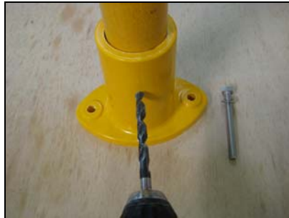
Drill through any base fittings with 8mm drill
