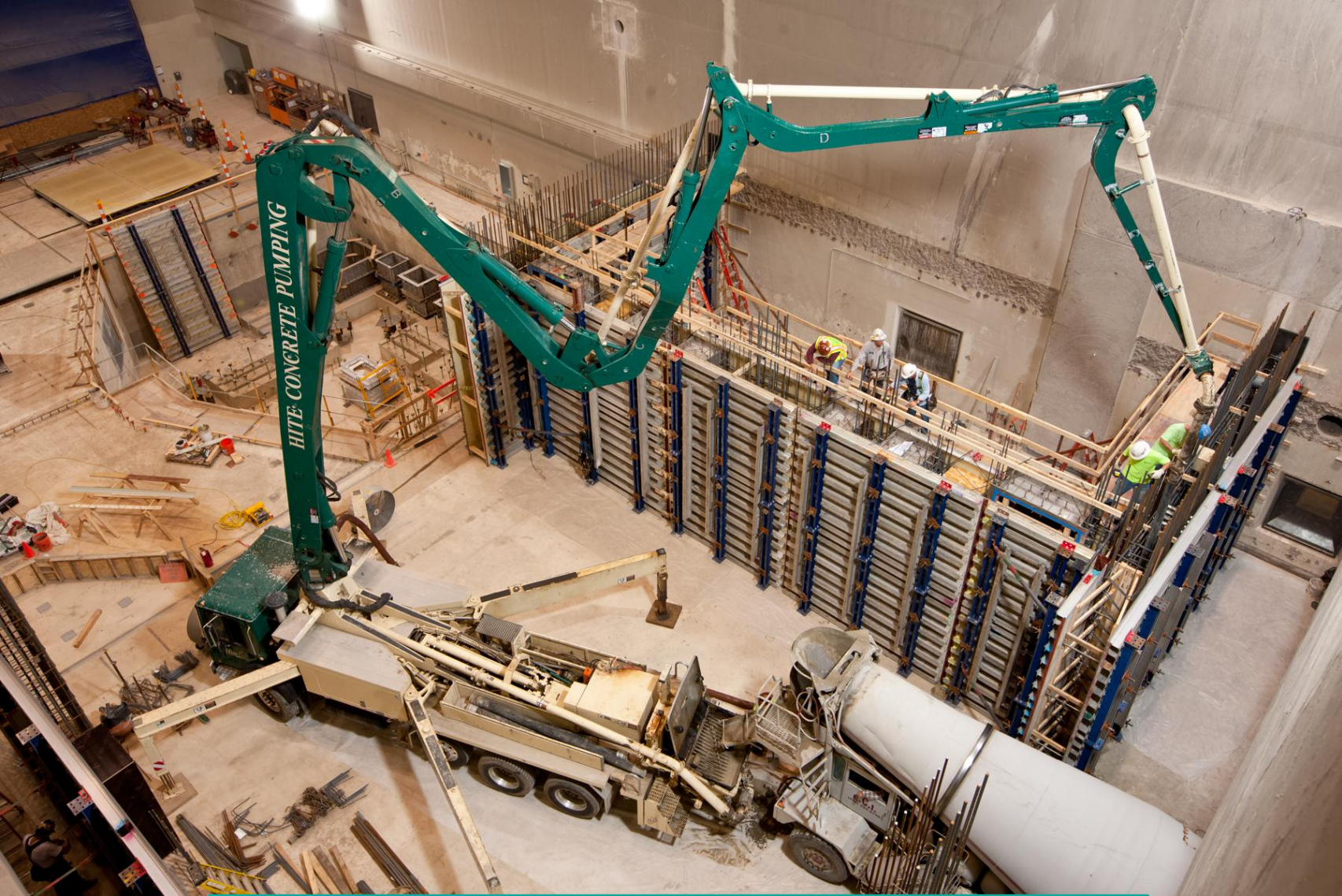
Concrete pour #1 completed October 2009
