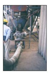
In July 2005, Zen-Noh Grain Corporation installed a DMN model AL300/3C hard chrome plated valve in the worst case location in the system. All these locations are open to the elements of nature, and after surviving both hurricane Katrina and Rita, this valve has run continuously without any downtime for repairs or replacement. Even the standard paint, as seen above, has weathered very well and shows no signs of deterioration, even after the hurricanes. The price of the DMN valves was \$5,800.
