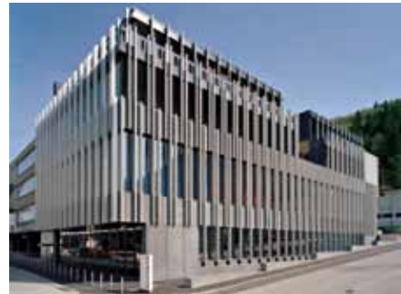
Built corporate identity. The facade of the corporate headquarters in Littau near Lucerne features vertical aluminium plaster strips that form an excellent point of reference with our products and market partners.
