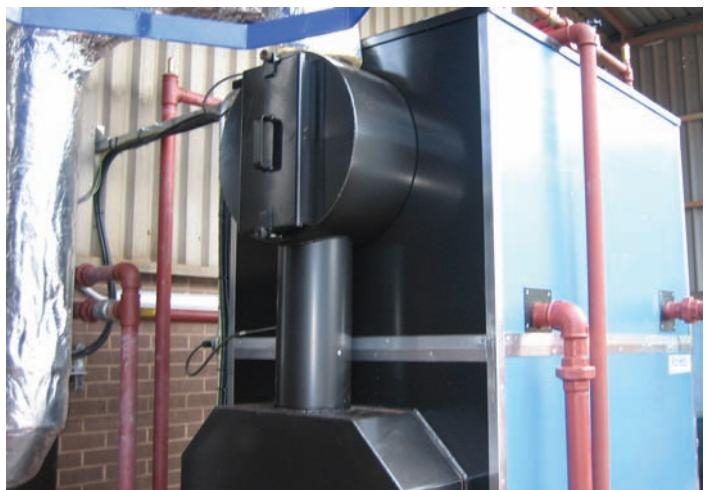
*Below: 150kW Ranheat boiler with economiser mounted on top*
