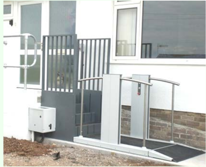
Lift with bridging steps
