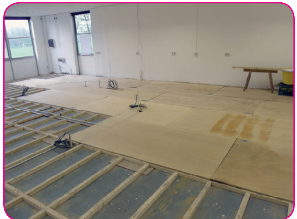
new floor which had to be installed
