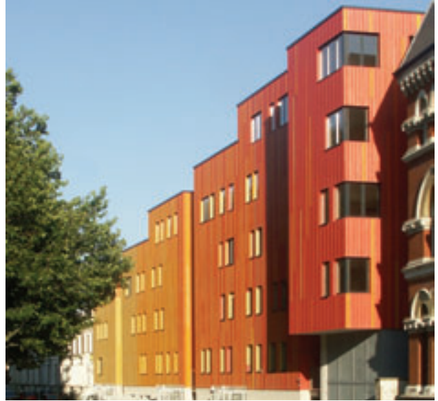
Cedral Weatherboard, Social Housing, Wansey Street, London
