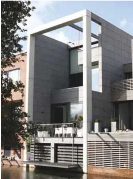
Private house | Architect: Beishuizen Ongerling Smets Architecten | Colour: Linen
