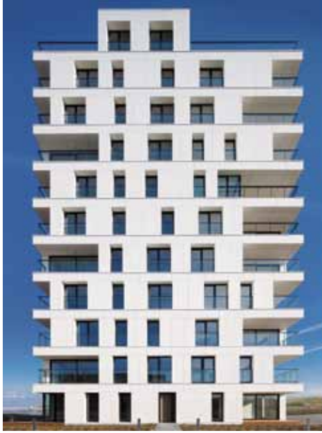
Apartment block | Architect: Botnick Architecture & Engineering | Colour: Calico
