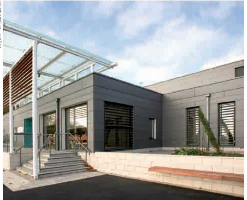
Singleton Hospital, Swansea
