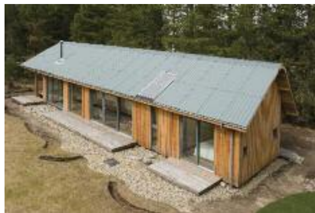
Tuath North, private residence using Profile 6
