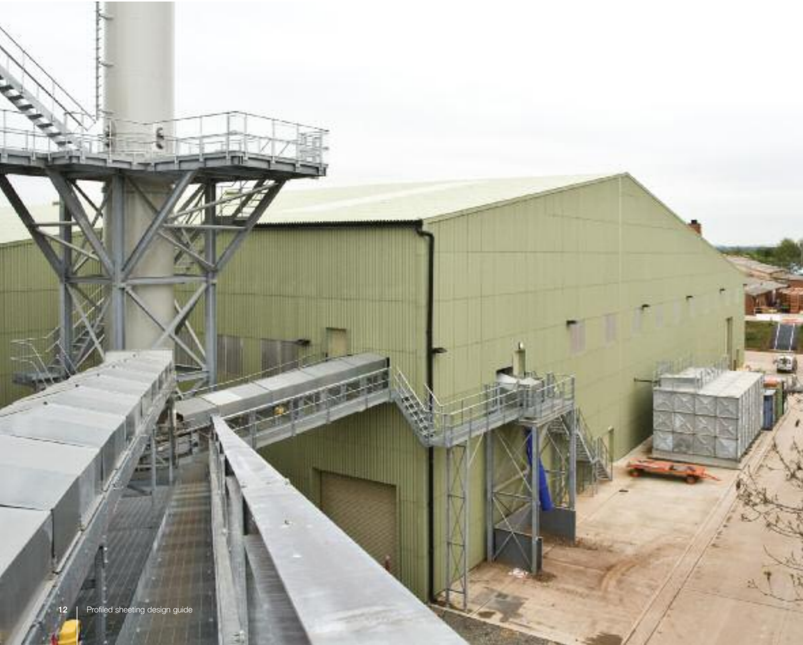
Hanson brick manufacturing plant, using Profile 6
