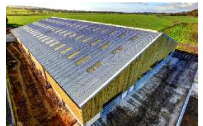
Ashdowne Grange Farm, using Profile 6 with spaced roof ventilation system
