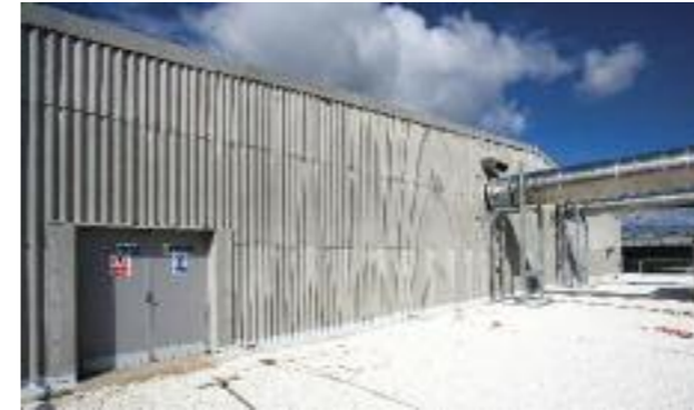
Wrexham Waste Disposal centre, using Profile 6
