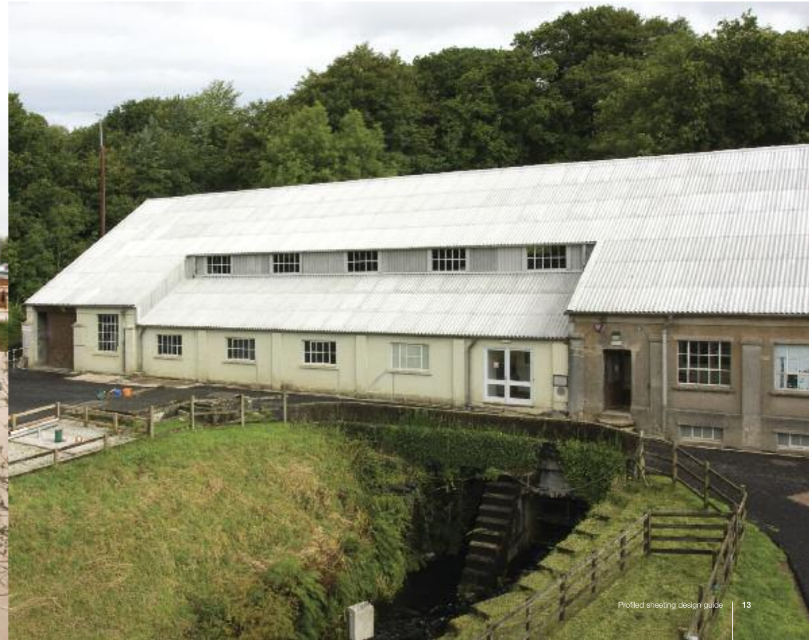
Mary Tavy hydro electric plant, using Profile 6
