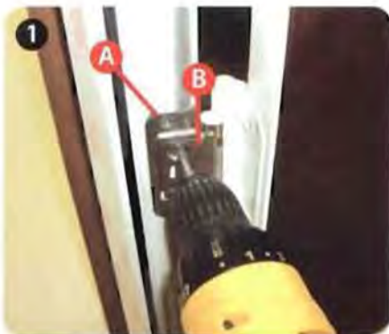
Remove the 2 screws that clamp side plate (B) to frame plate (A) to all three hinges
