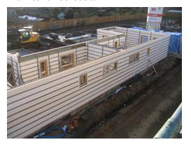
Polarwall was constructed off a concrete strip foundation utilising the Hanson Jetfloor for the ground floor structure and open web joist floors for the first floor. Standard roof trusses were also used.
