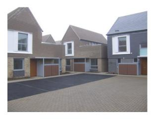
The 2 story buildings have been completed to provide a variety of occupancy dwellings. Cladding is a mixture of a conventional masonry, rendered sections and tile hanging to interact with the local vernacular.
