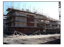
A mixture of 2 and 3 stories has been completed to provide a variety of dwellings. Cladding is a mixture of a conventional masonry skin and render.
