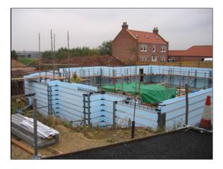
The ground conditions were such that the basement had to withstand significant hydrostatic pressures. Thus the design specification for the formwork provided for a 300mm concrete core with a single mesh of T16 reinforcing steel. The polystyrene shutter utilised the XPS grade given its excellent mechanical and moisture resisting properties. This also provided a U-Value of 0.27W/m2K, ensuring compliance with Part L of the Building Regulations.
