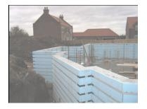
Key facts Core size Basement 302mm Insulation Standard 0.27Wm<sup>2</sup>K
