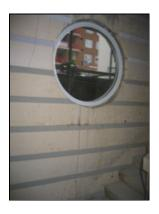
Polarwall was used to provide a cost effective method of construction with built in energy performance to a U value level within the walls of 0.27W/m<sup>2</sup>K.
