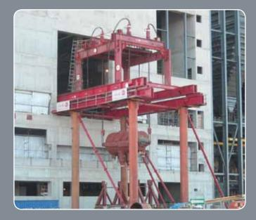
**OVERVIEW**: ALE completed a series of successful installations of heaters and a feedwater tank at the Wilhelmshaven power plant.
