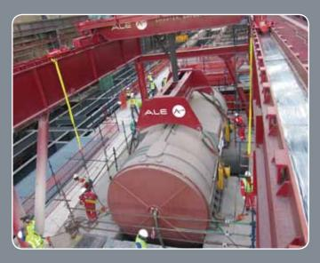
**OVERVIEW**: ALE successfully transported and installed six 360te stator generators for the Medupi power station and six stator generators for the Kusike Power Station.
