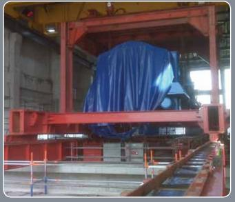
the longitudinal skidding operations were completed, each item was jacked up with the use of a hydraulic jacking system. A transversal skid system was then installed to position the heaters above their final foundation, from where they were jacked down by the hydraulic jacking system and installed.
