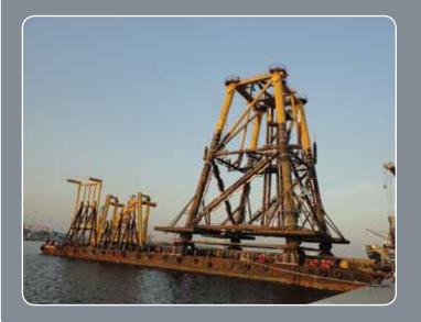
**OVERVIEW:** ALE successfully completed the transportation and load-out of piles and a jacket weighing 197te and 1,012te.
