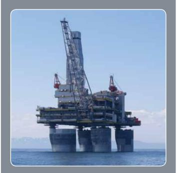
**OVERVIEW:** ALE provided the engineering, equipment and offshore management of the high capacity barge ballast system required for two of the world's heaviest floatover installations, weighing 28,000te and 32,000te.
