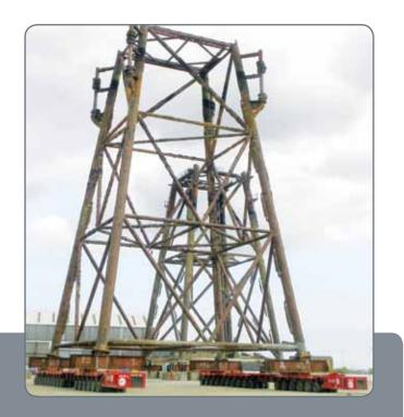
**SERVICES REQUIRED:** ALE have successfully completed the load-in and site movement of the jackets weighing between 800te and 1600te, the topsides weighing between 400te and 1,200te and the bridge weighing 80te. The loadins were undertaken using various different combinations of SPMTs with a maximum of 56 axles on site at any one time. ALE also provided the barge mooring and ballasting operations for each load-in.
