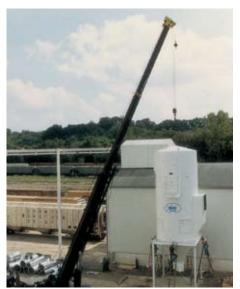
MCF Filters can be shipped fully welded to simplify and speed installation.
