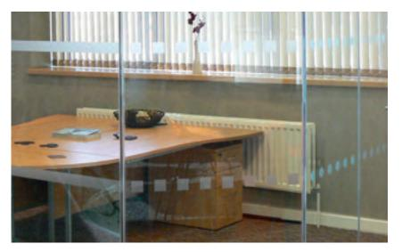
Film applied to meet the requirements of Part M of the Building Regulations
