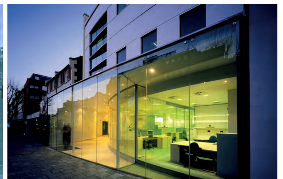
Top Left: Overhead glazing on primary steelwork. Top Right: Underlit laminated glass floor panels with sandblast finish. Above & Left: Bespoke glass entrance and facade on glass fin supports.
