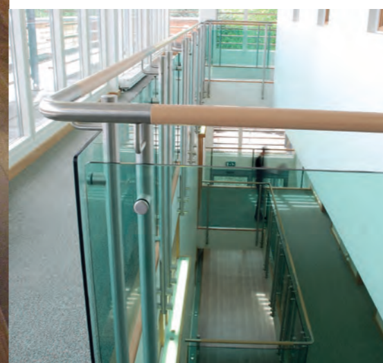
Above: Timber and stainless steel balustrade with glass infill.
