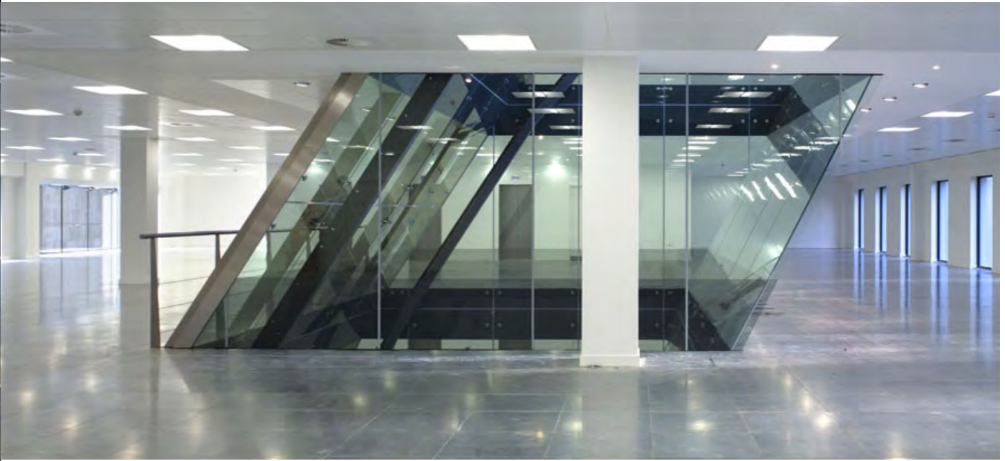
Centre Left: Modern glass link bridge complements traditional structure. Centre Right: Curved and faceted 2 edge supported glazing. Bottom: Structural glass feature doubles as a central atrium.
