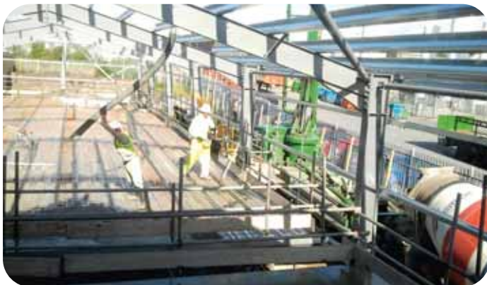
Concrete for the upper floor is pumped in from a truck.
