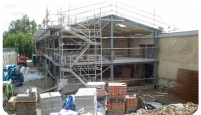
With the concreting finished work commences on the outer walls.
