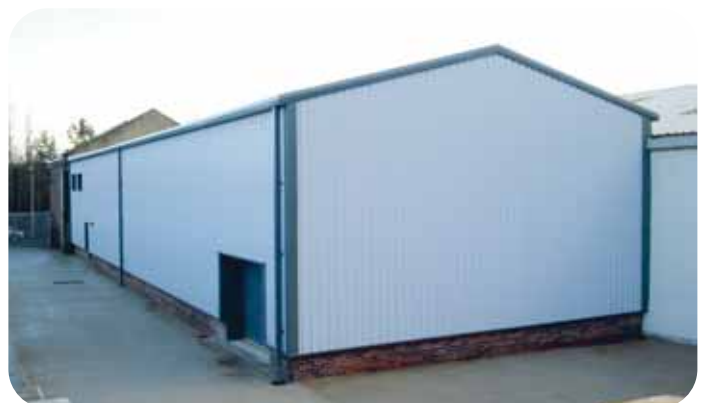
Our 2 storey, 600 square metre, extension is complete. It provides us with extra manufacturing, warehousing and office space.
