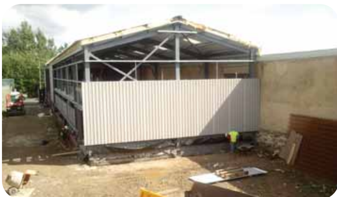
Cladding and roofing work continues.
