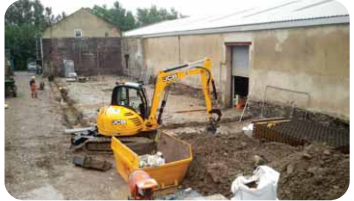
The cleared site is prepared for steel works to be erected.
