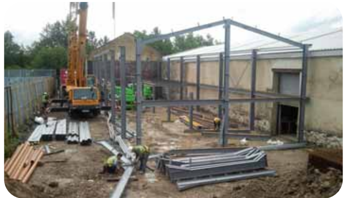
The steel frame quickly takes shape.
