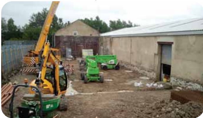
With concrete pads in place the steel frame can be assembled.
