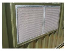
Stainless steel salt filters protect the equipment in coastal locations.
