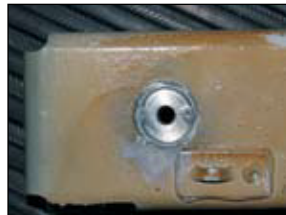
Hole prepared by a typical wire brush demonstrating terrible overall surface contact.
