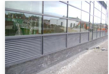
Penthouse Turrets and Weather Louvres at the College
