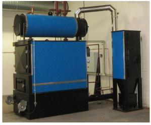
exhaust flue gasses from a boiler and then passes them through another two passes in a heat exchanger to extract more of the heat from the flue gasses. The flue temperature typically reduces by over 100°C giving the increased efficiency. Economisers
