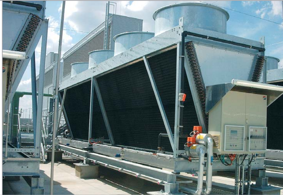
Hybrid cooler for data center
